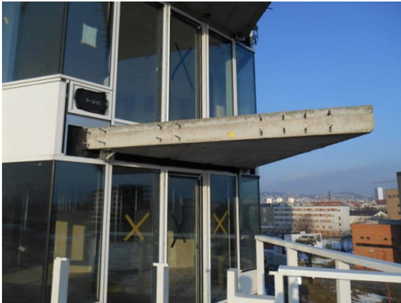
balcony – Tower 1 SW facade
